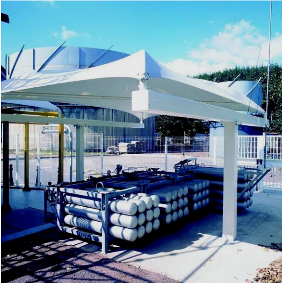
Picture 8. Biogas fuel storage unit at Marquette
