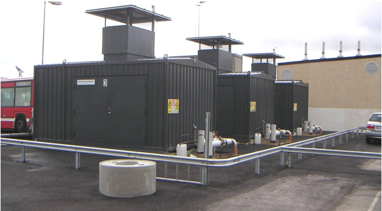
Picture 4. Bus depot with three compressors and 350 bar CBG storage
