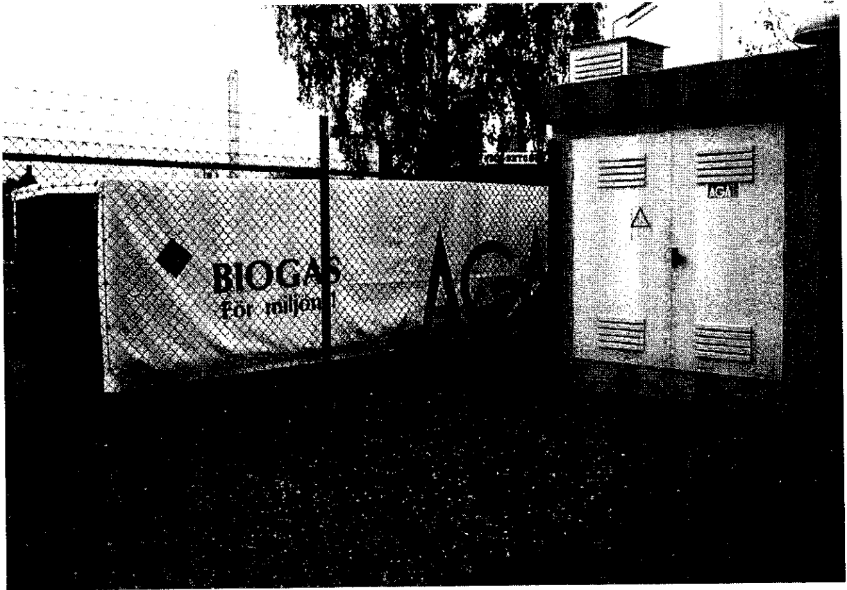
Figure 5. Gas Platform. Containing 1.900 Nm 3 biogas
